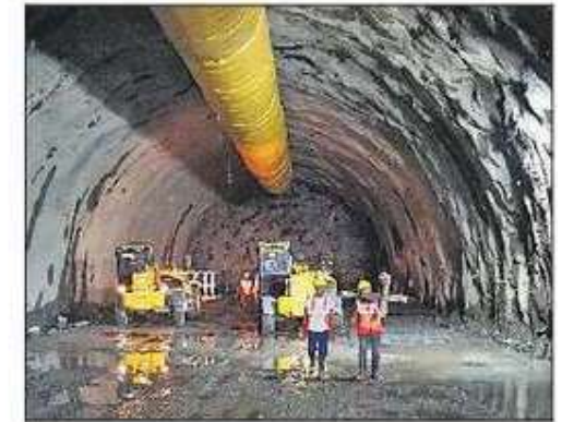
Work in progress near Ghansoli. PRAFUL GANGURDE /HT
